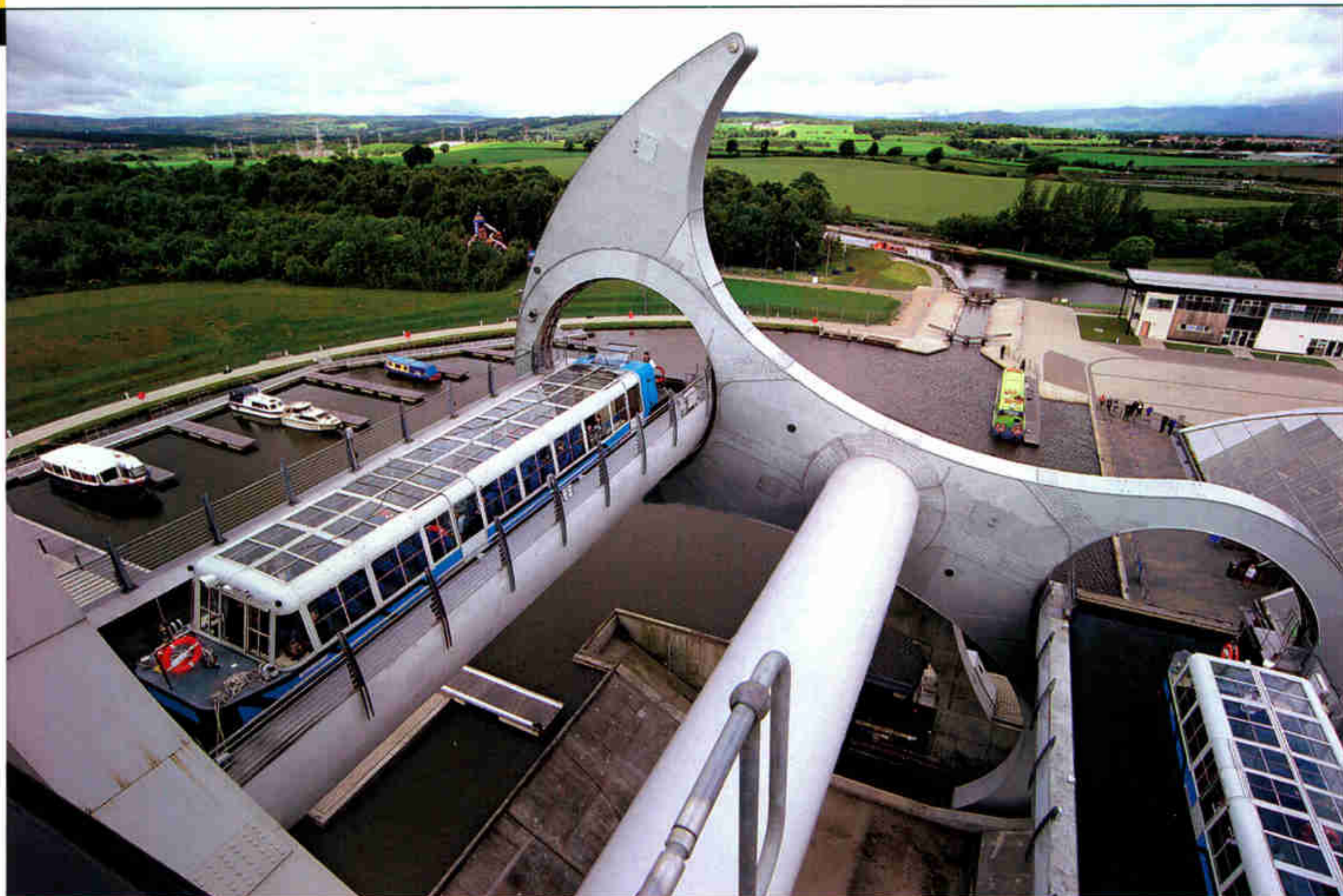
A streamlined substitute for 19th-century locks, the Falkirk Wheel near Falkirk, Scotland, transports boats up and down a steep drop, linking two major canals for the first time in almost 70 years.
